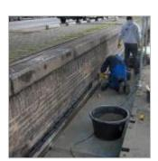
The expansion joints on the crosscut edges must be at least 1 cm wide to allow for the expansion of KLP<sup>®</sup>. This joint can be sealed.
