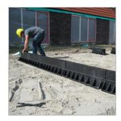
KLP® Foundation Blocks are designed for lightweight structures such as storage and garden sheds. The easy-to-place plastic foundation blocks offer many advantages over the alternatives from concrete and wood. Seven reasons to choose KLP® Foundation Blocks:
