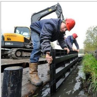
The panels are tough enough and stiff enough to be pushed into soil by crane. The KLP® RapidRetain panel coupling is made strong, so that no pole is needed directly in front of each connection. The result is that all poles can be placed in one go and subsequently the panels can be placed in one go, which translates to faster turnaround times and therefore savings.
