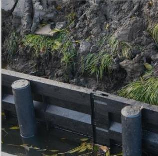
**KLP® RapidRetain System** presents a sustainable and cost efficient solution for your retaining wall! KLP® plastic is an excellent choice, especially at the water and air interface, where wood is most sensitive to rot. KLP® RapidRetain system consists of KLP® RapidRetain panels and KLP® RapidRetain combi-poles.
