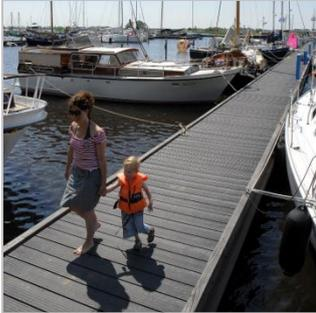
Landing stages and jetties made from recycled **KLP® Deck** have the charm and usability of wood plus the durability of plastics. The material has an expected technical lifetime of at least 50 years and is maintenance free. Calculated over the whole technical lifespan, you are better off financially with KLP®. With the following parts you can construct a KLP® Landing:
