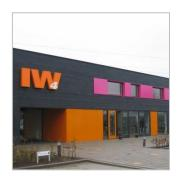
KLP® Façade panels can be applied on office or school buildings, houses, sheds and garden partitions. Both horizontal and vertical mounting is possible. The panels are mounted by means of an aluminium H profile which not only provides invisible fixing, but will also allow for natural expansion and contraction.
