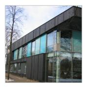
Due to the material's properties the facades have a very special appearance. This is emphasised even more by using anthracite-black planks and by the surface structure of KLP<sup>®</sup>. The fibre structure of KLP<sup>®</sup> gives depth to the plank thus giving it a natural appearance.
