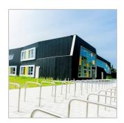
The panels are produced from recycled, polyolefin plastics. KLP<sup>®</sup> has the charm and usability of wood and the lifespan of plastics.
